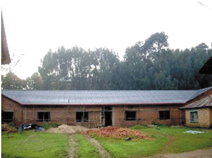
Rwankeri School New Dormitory.
