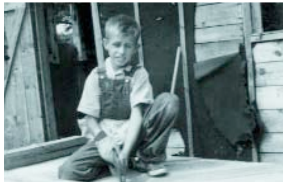
Figure 7. 1954 – Early training in house building.
